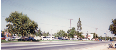
Commercial uses along Van Buren Boulevard
