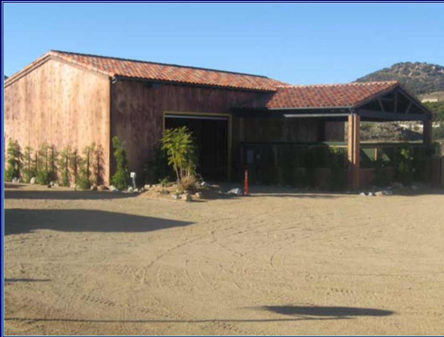
side of the accessory structure
