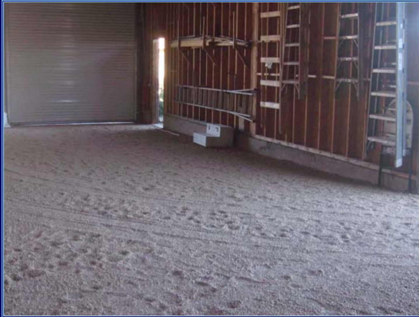
Inside the accessory structure
