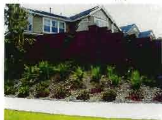
MASONRY BLOCK WALL
