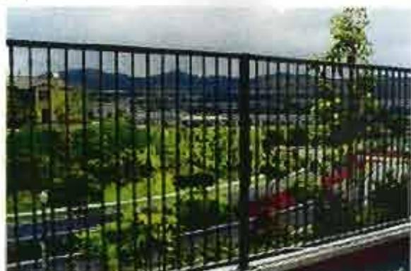
TUBULAR STEEL FENCING AND / OR COMBINATION BLOCK WALL AND TUBULAR STEEL COMBINATION VIEW FENCE.
